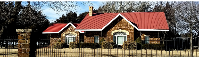
George Eschbaugh Studio constructed from Dakota Sandstone from the Wilson Depot which was constructed from the stone from the Fort Harker Military Hospital.
